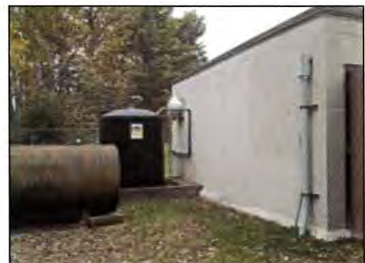
Woodland Manor Pump Station
