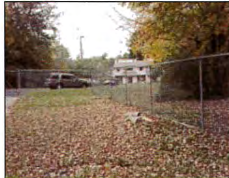
Pump Station Fencing
