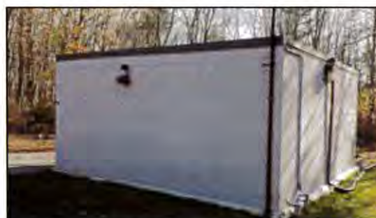
P.S. Building Lighting / Alarm
