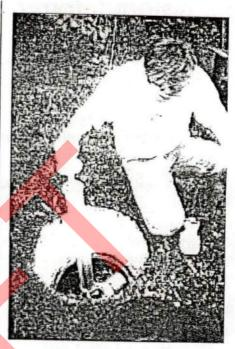
An effluent filter, installed at the outlet end of the septic tank, is easily maintained when an access riser is installed to grade on the septic tank.
