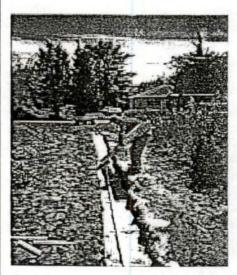
The shallow, narrow drainfield design is a typical component of the enhanced treatment system.
