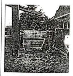
The seam of this concrete septic tank is sealed with a butyl strip that provides additional assurance that is waterlight. The inlet and outlet have cost in place rubber boots with stainless steel damps.
