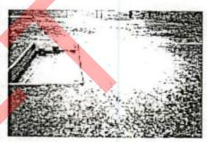
Purt of this single pass sand filter is exposed at URI's On Site Wasterwater Training Center for demonstration purposes it is one example of an enhanced treatment component approved for use in Phode I sland.
