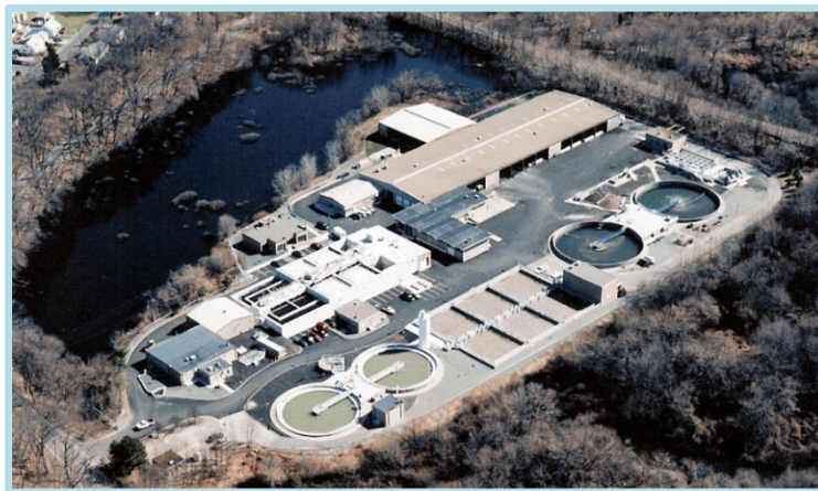
West Warwick Regional Wastewater Treatment Facility
