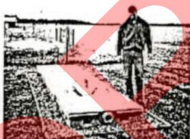
Flow diffusers are another conventional drainfield option. Installed in crushed stone and finished with 18" of topsoil and planted in grass.
