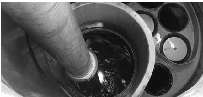
Vacuuming Sump Through MAW
