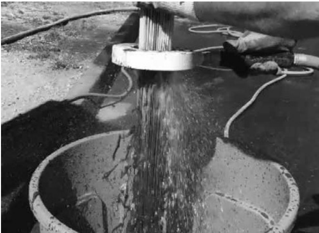
Rinsing Cartridge with Contech Rinse Tool
